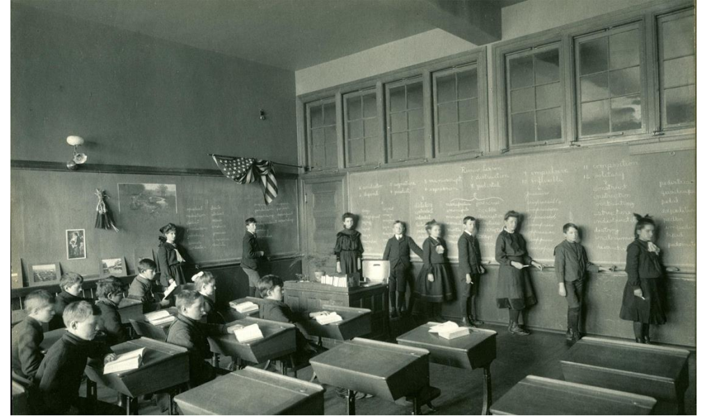
HORACE MANN INTERIOR (HISTORIC) PHOTO FROM SULLIVAN BUILDING
