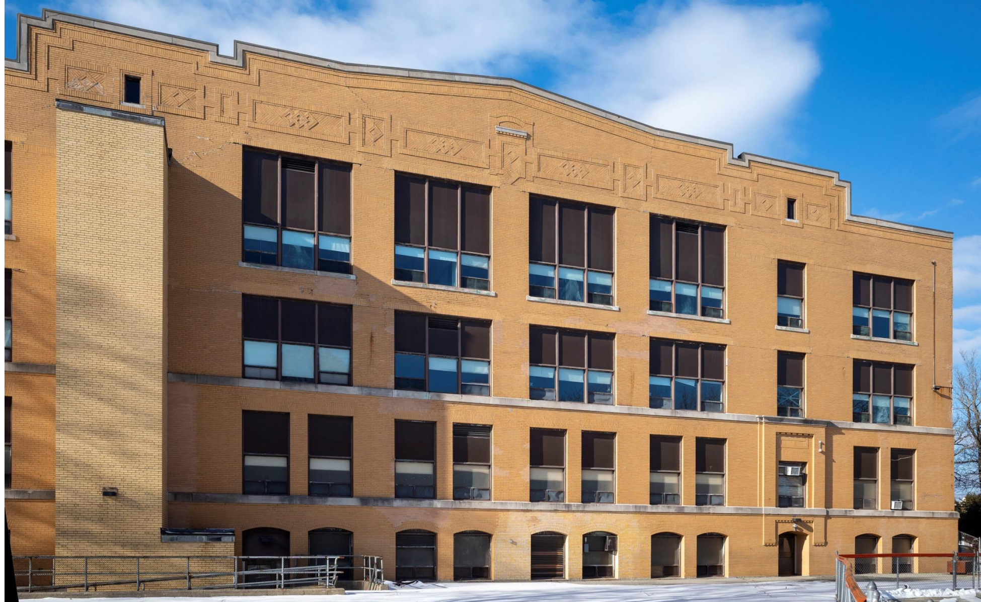
Campus Side Existing Building
